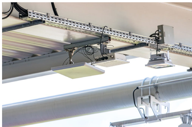
Outdoor access point LANCOM OX-6400 with sector antenna AirLancer ON-Q30: positioned high up in the stadium roof, this combination ensures comprehensive and powerful Wi-Fi coverage on the stands of the Heinz-Steyer-Stadion. Image rights: Sandra Hofmann
