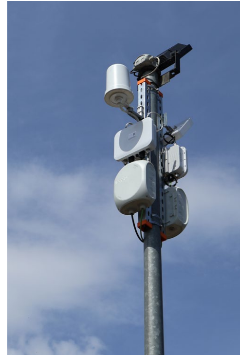
Image source: M. Busch, outdoor area coverage – outdoor access point LANCOM OW-602 with outdoor omnidirectional antenna featuring a 360° beam angle
